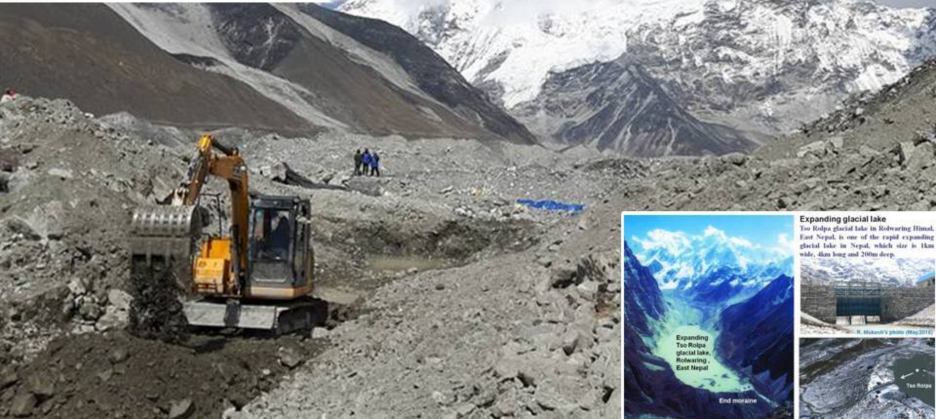
Artificial canal (Google Image: 2008.11.21) An artificial canal (red mark) was constructed at the terminal moraine of Too Rolpa to lower the water level.
